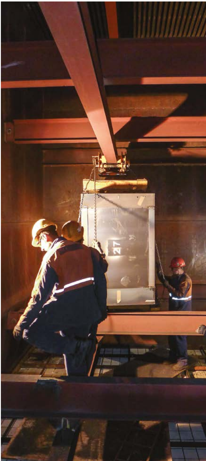
↑ Installation of Modules to SCR Reactor
