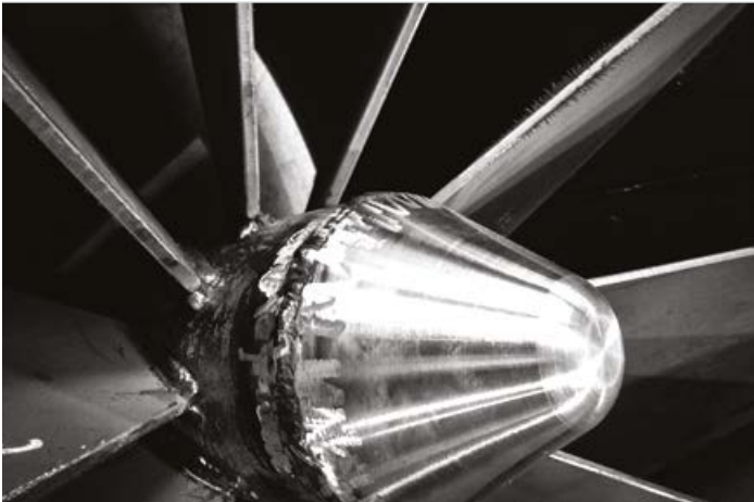
↑ Fly Ash Separator in the Flue Gas Duct
