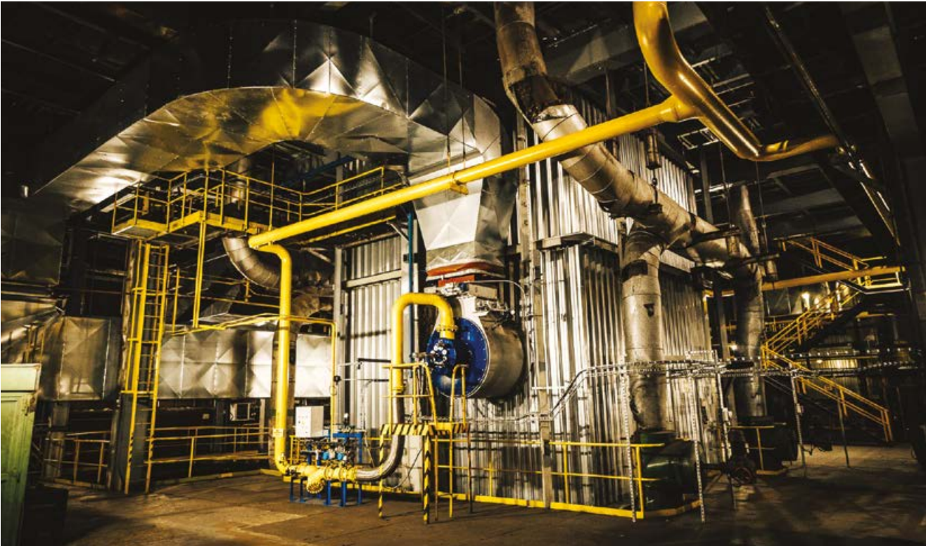
↑ Gas Hot Water Boiler 116 MWt
